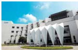
Tainan Plant (Diamond-rated Green Building)
